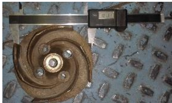
Figure 3: View of the pump's impeller
